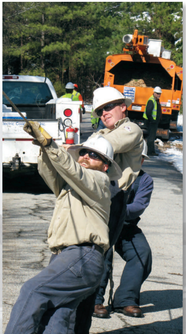
LINE CREWS WORK IN TREACHEROUS CONDITIONS YEAR-ROUND TO RESTORE POWER WHEN CONDITIONS CREATE OUTAGES
